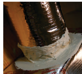
Mastic Sealed Round Duct
